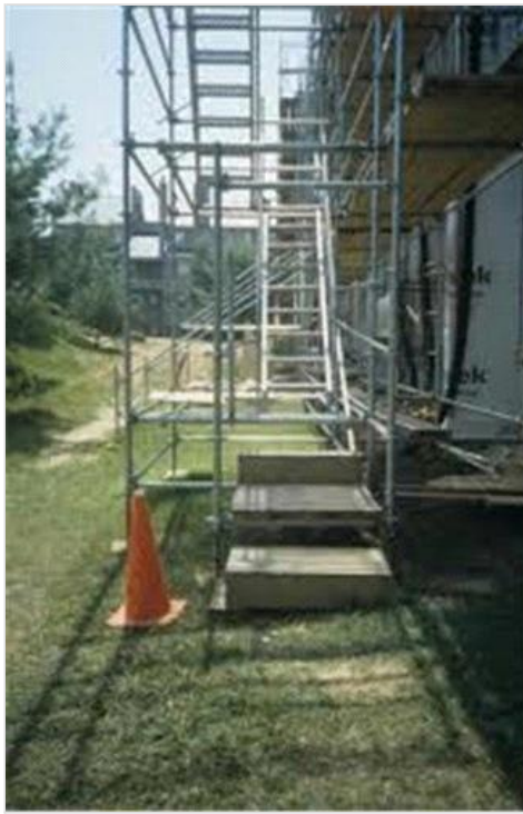
Scaffold at Rear
